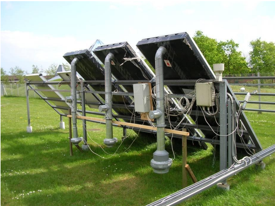
Fig.3 Photo of the mounted PVT collectors
