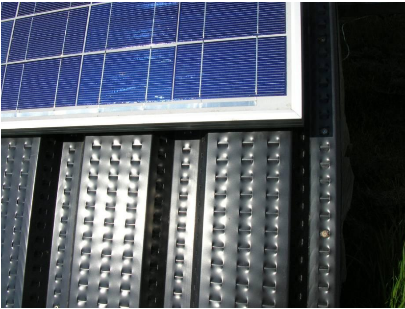
Fig.4 The frame of the PV modules are mounted directly on the SolarWall element. Air is transpired through all the small holes in the black metal profile.
