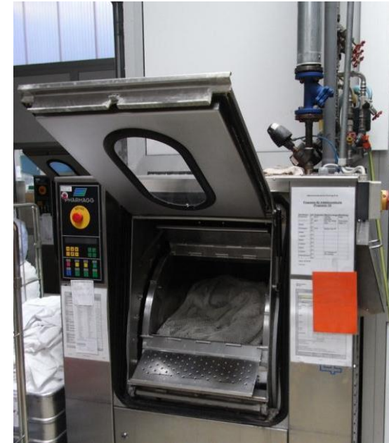
Industrial washing machine with hot / cold water and steam connection
