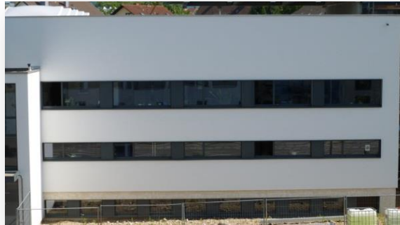
Façade facing street - After retrofit.
