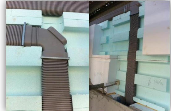
Second 140mm layer insulation covering airducts
