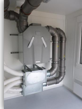
Below: duct connection to the air handling unit in container
