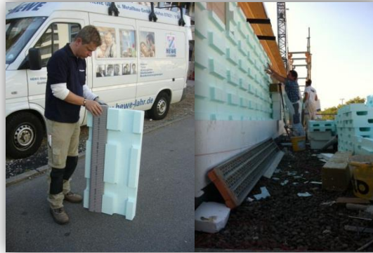
First 100 mm layer insulation with air ducts
