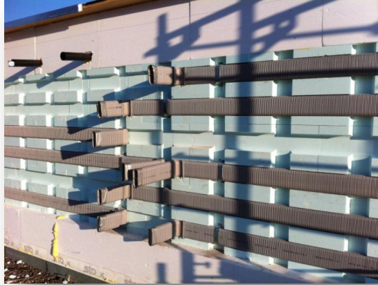
Above: Ventilation ducts refab window frame with air inlets/outlets on top
