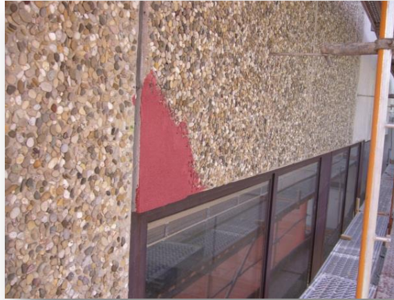
Façade detail - Before retrofit.
