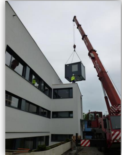
Above: container with air handling unit
