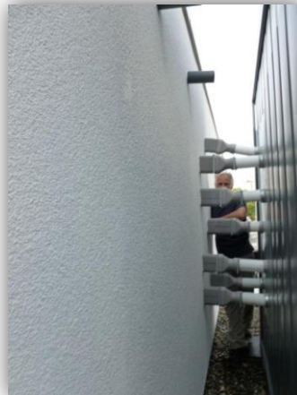
Below: duct connection to the air handling unit in container
