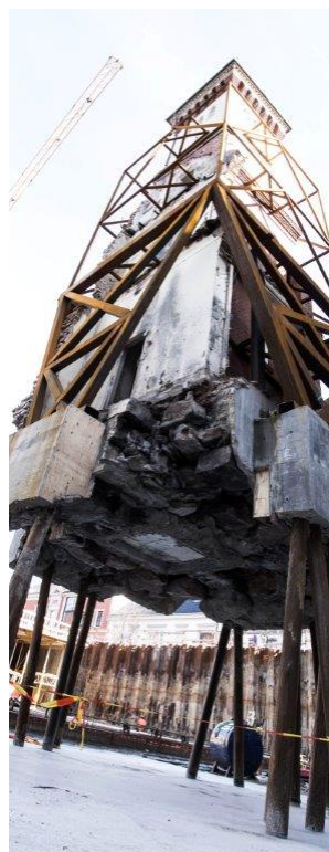
Photo: The old fire tower, Strømme
