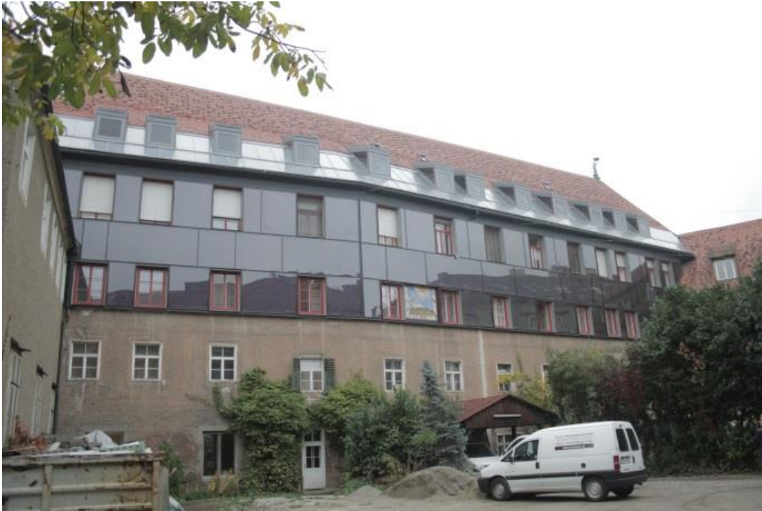
(Gebetsroither A.) Southern wing of the monastery with solar thermal façade / roof
