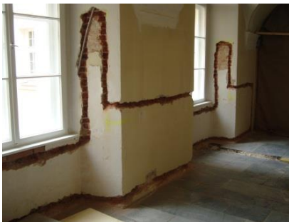
(Knotzer A.) Installation of component heating
