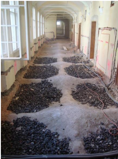
(Knotzer A.) Insulation with foam glass gravel in the floor
