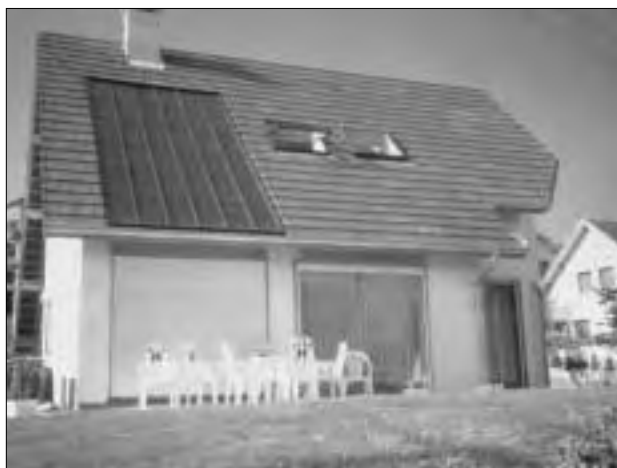
Figure 4. French house equipped with a direct solar floor system (Source: Clipsol, France)
