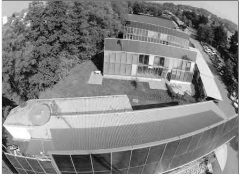
Figure 10. 60% of the space heating demand of these terraced houses are covered by solar energy (Source: AEE INTEC, Austria)
