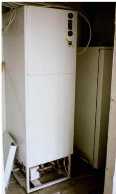
The system uses a standard solar domestic hot water tank with all components of the system integrated in the same cabinet as the tank. The dimensions of the cabinet are furthermore modular 0.6 x 0.6 m, so that it easily fits into the utility room.
