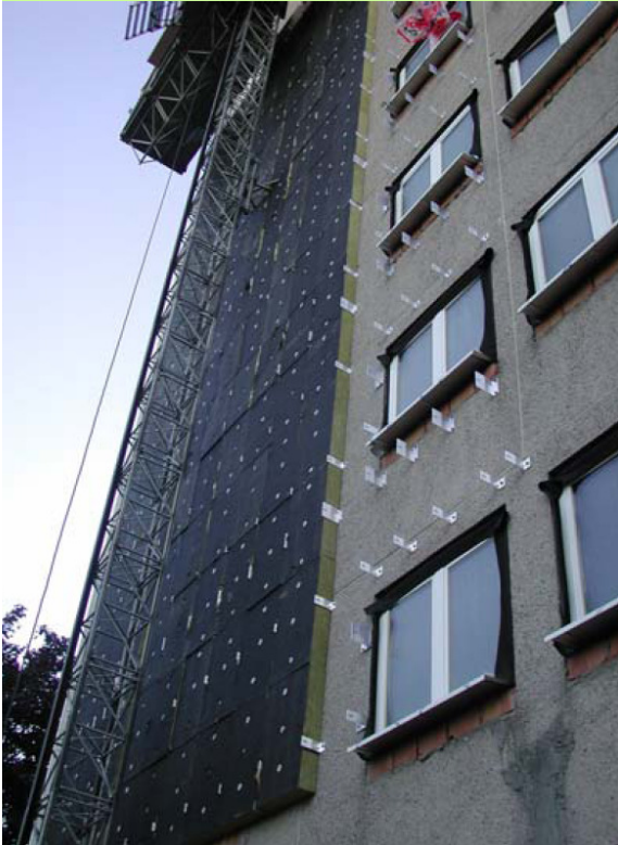
Mineral wool insulation being installed on the existing concrete walls of the north façade.
