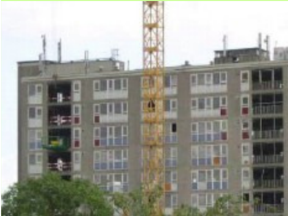
The old apartment block being stripped.
