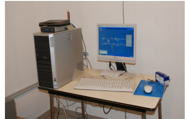
The central monitoring system for the buildings Zonneveld and Sterrenveld.
