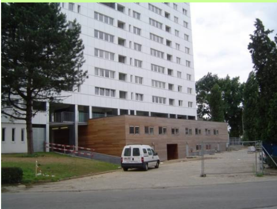
The new residences on ground floor, and the storage rooms on the first floor: above on the west façade and below on the east façade.
