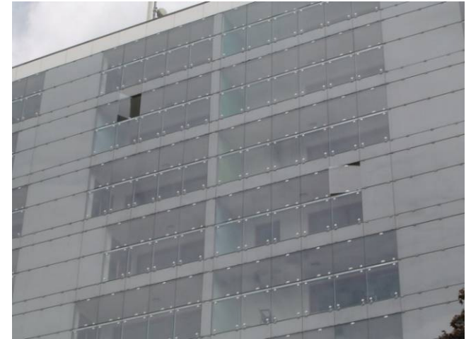
The new winter gardens. It is possible to open the glazing and so to have a normal balcony.
