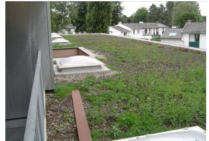
Green roof on top of the new residences. In the background you see the single family housing of the garden city.
