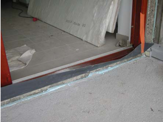
Thermally insulated connection between winter gardens and concrete structure.
