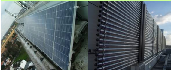
photovoltaic solar panels and vacuum tube solar heating system on the roof of Sterrenveld.
