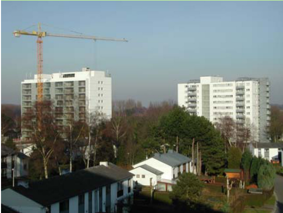
An aerial view of the garden city Ban Eik. In the middle you see the two apartment buildings, Sterrenveld to the left and Zonneveld to the right.
