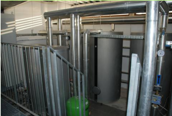
The 2 300l buffer tanks in front, and the 3 1000l buffer tanks in the back.
