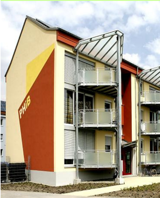
Reduction of thermal bridges by erecting stand-alone balconies in front of the facades
