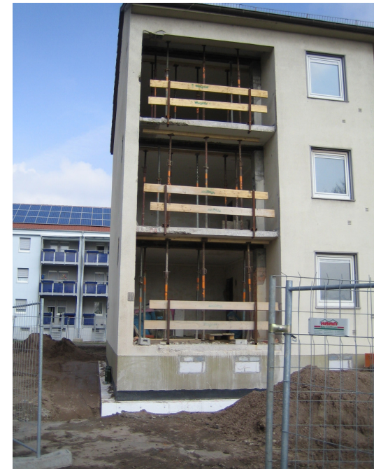
Removal of the existing balconies - one of the greatest thermal bridges
