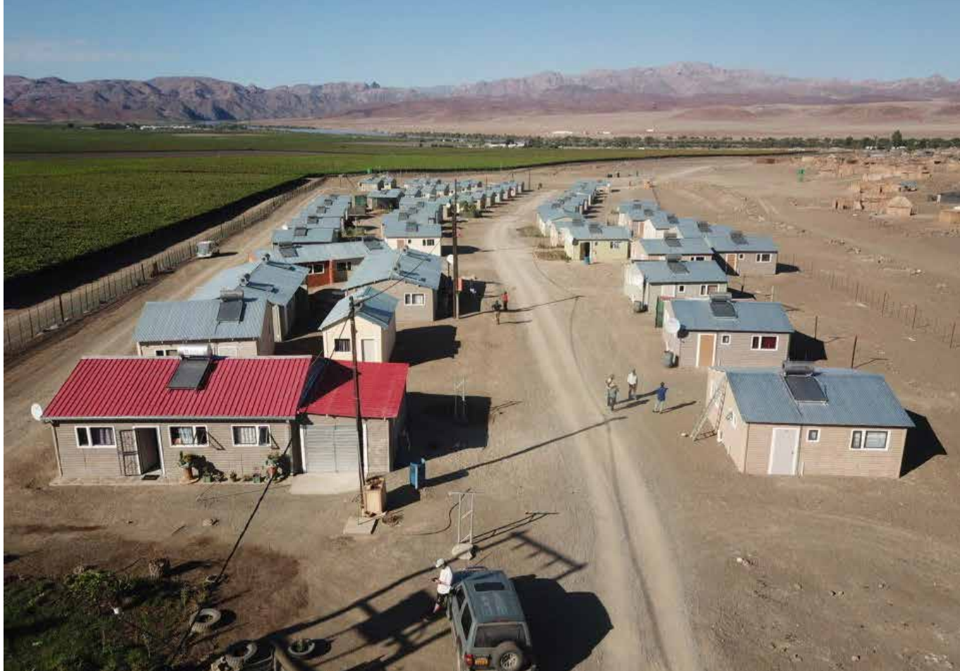
NOBLE PROJECT ... The Orange River Vineyards Investment (ORVI) social housing project which is this year's the winner of the International Energy Agency Solar Heating and Cooling Programme Solar Award
