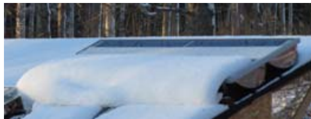
Fig.4 Ice Dam Formation on the PV Integrated Roof Mock-up.
