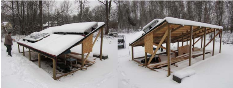
Fig.1 PV/T HR Roof System Mock-up Built by Finsun Inresol in Alvkarleby, Sweden.
