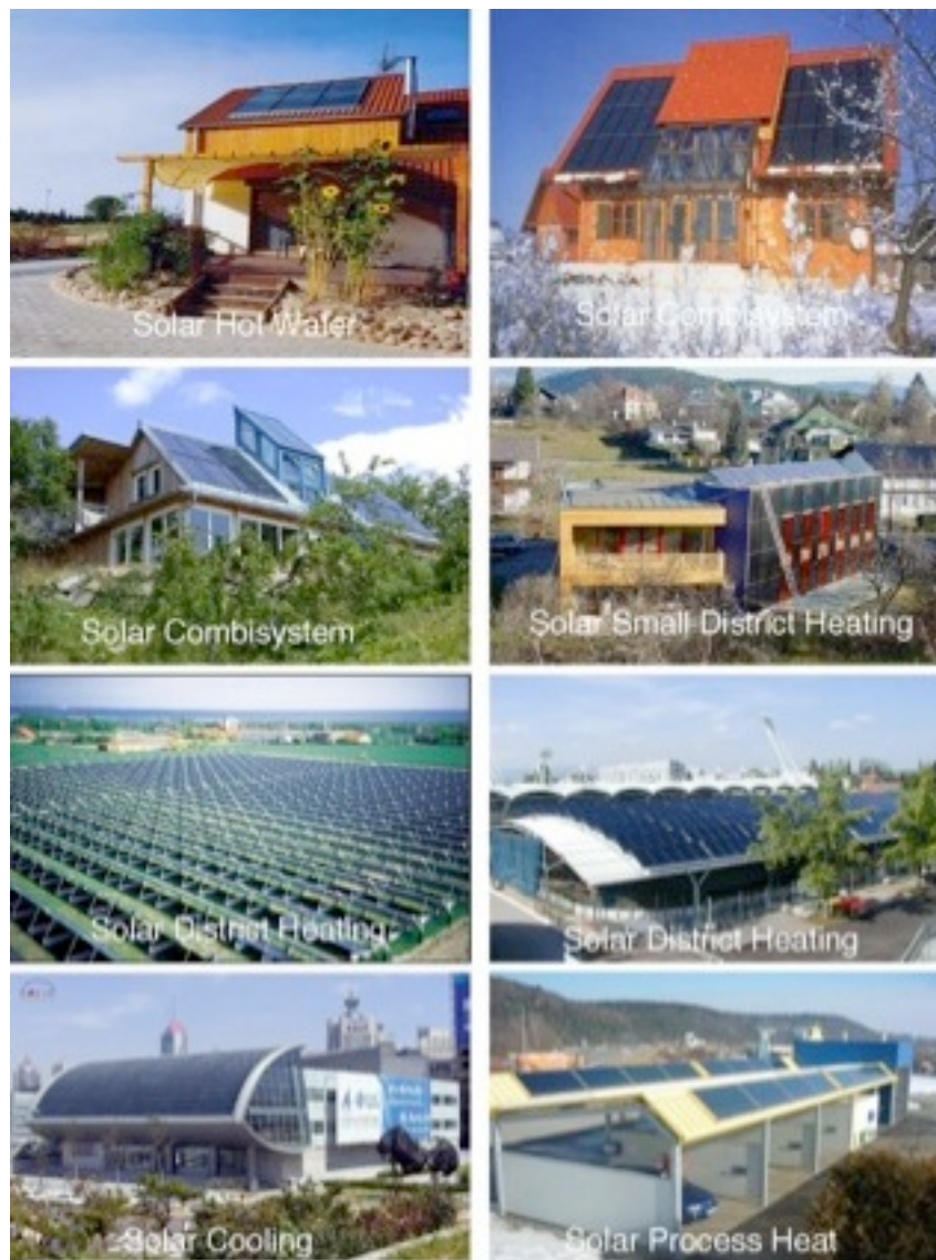
Figure 2.2. Solar thermal systems for low to medium heat production.
