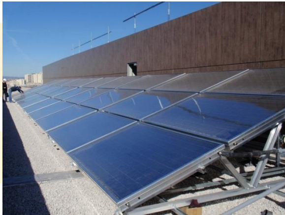
Picture of the collector field
