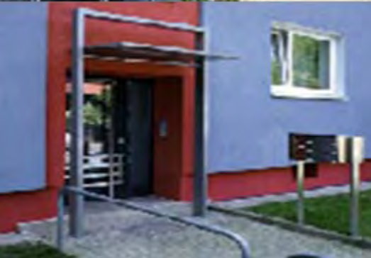
Views of new balconies and entry
