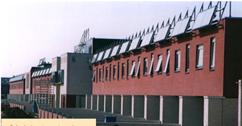
Solar hot water systems in the Apeldoorn solar project, the Netherlands (Source: Ecofys, NL-Utrecht).
