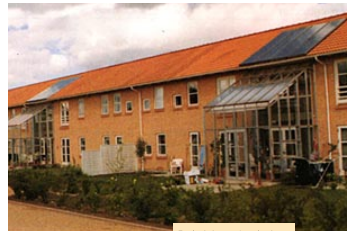
Typical domestic solar hot water systems in Denmark.
