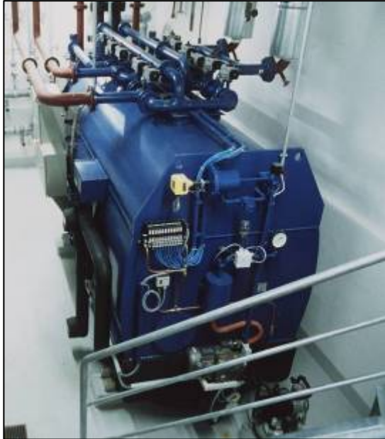
Nishiyodo NAK 70 kW capacity
