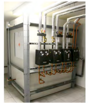
FLEXSAVE VARIO: Modular buffer storage with polymeric liner for residential buildings
