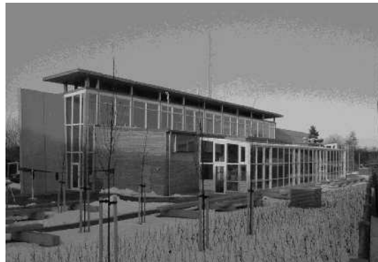
Community Centre in Kolding, Denmark (Photograph by Municipality of Kolding)
