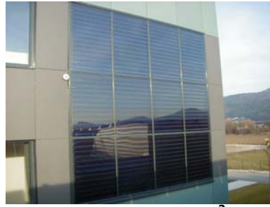
Test façade with a 25 m 2 collector on an office building in St. Veit, Austria.
