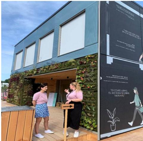
The energy concept of the LOCAL+ team from the University of Applied Sciences in Aachen, Germany, uses façade-integrated PV elements (blue on the photo). These are color coordinated with the other building materials to increase the acceptance of onsite energy production.
