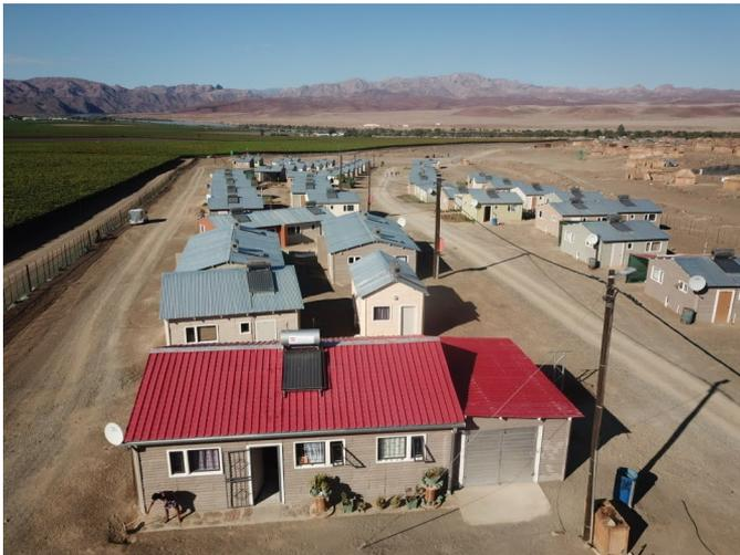
traditional reed huts, which do not have water, sanitary facilities, and electricity connections. To provide farmworkers with affordable yet sustainable and energy-efficient homes, ORVI, one of the Orange River Vineyards, developed a housing project to accommodate its employees. It comprises 58 houses made of precast concrete bricks, with pitched roofs and ceilings, all built during 2020. The houses all have potable water and an electricity connection.
