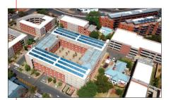
▲ University of the Witwatersrand Junction Student Residences uses a pumped solar thermal system with a hot water storage tank and external heat exchanger. In one year, this installation gives a solar yield of 397.70 MWh and is responsible for avoiding 137,600 kilograms of CO, emissions. Source: SOLTRAIN
