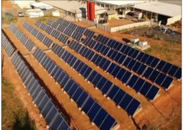
Klein Karoo International (Pty) Ltd Tannery (KKI) installed a solar thermal plant. In one year, this solar installation generates 397 MWh and is responsible for avoiding 137,000 kilograms of CO, emissions. Source: SOLTRAIN
