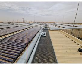
Solar cooling system at Camp Castor in Mali. The system uses 700 m2 of vacuum tube solar collectors to drive an absorption chiller with a 348 kW cooling capacity to provide AC to a cafeteria and kitchen. Photo credit: Frank Molter, **SolarNext**
