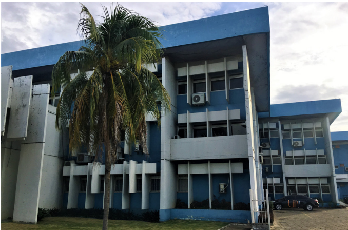
Figure 2. Forum Sobral Pinto, Northeast Façade.
