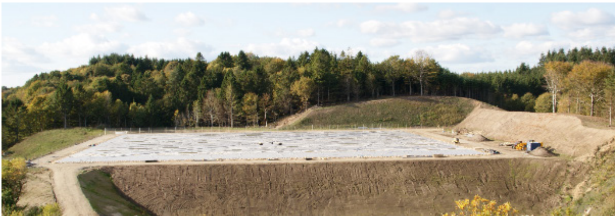
Figure 6: Water pit storage at Dronninglund Fjernvarme. Source: Dronninglund Fjernvarme
