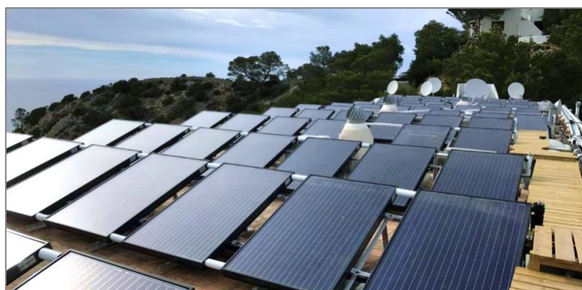
A PVT field of collectors on a flat roof is not different from a T field or a PV array. Integrated solutions will look totally similar to PV-only solutions. Credit: Endef - Spain
