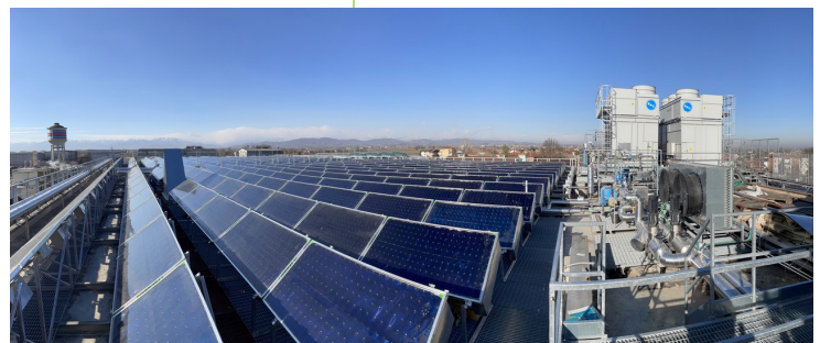
▲ Solar process heat system for Martini & Rossi, with a capacity of 0.42 MWth, is equipped with high-vacuum flat plate collectors, Turin, Italy. Photo: TVP Solar, Switzerland.
