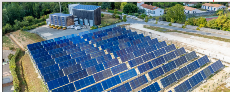
◀ Panoramic view of the Pons solar thermal system. Source: Newheat
