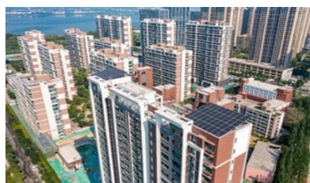
Residential solar engineering in Taiyuan, Shanxi Province
