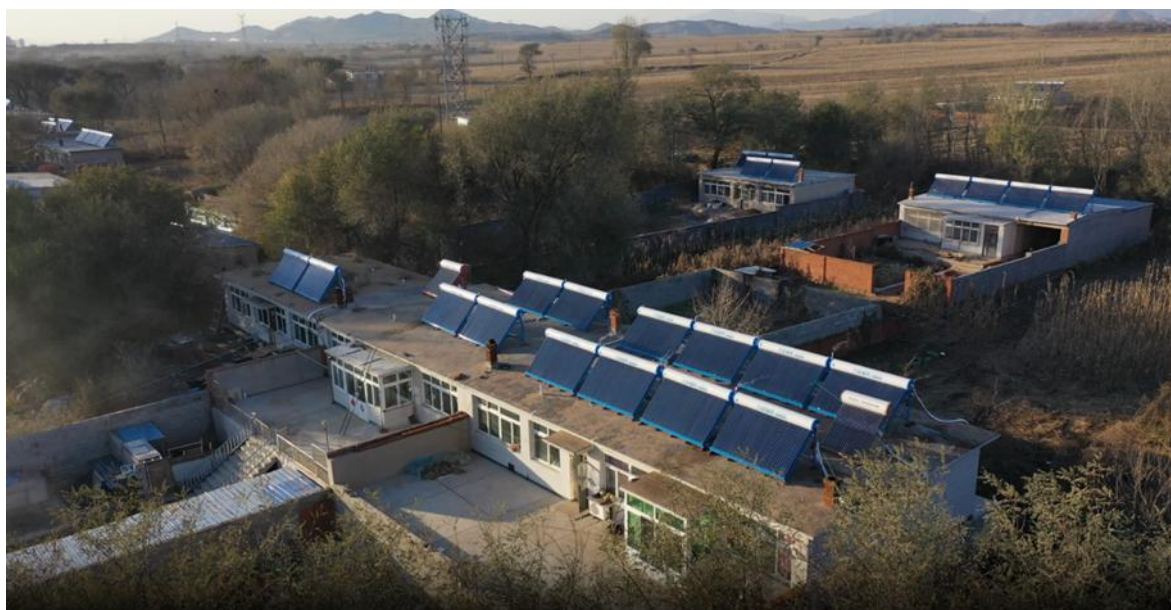
Figure 7. Huludao City Ecological Environment Bureau Longgang Sub-bureau Clean Heating Project, Liaoning Province, China. Source: Shandong Linuo Ritter New Energy Co., Ltd
