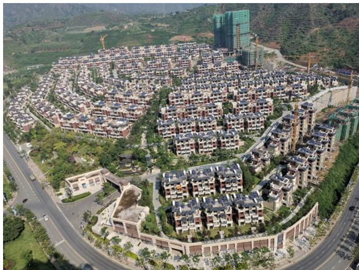
Figure 5. Puda Health and Wellness Resort, Panzhihua, Sichuan Province, China. Source: Shandong Linuo Ritter New Energy Co., Ltd
