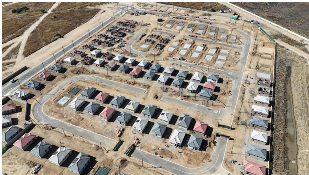
Figure 30. First phase of Tanganani affordable housing development under construction. Solar PV panels are visible on the roofs.
