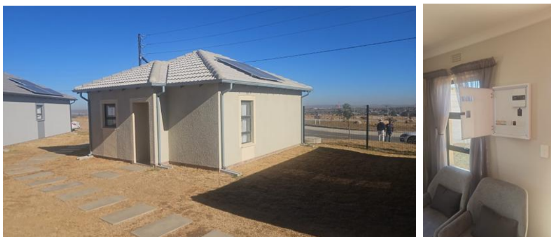
Figure 31. Example 2-bedroom house with solar PV panels (left), distribution board inside the 2-bedroom house with solar PV water heating control dial and USB device charging ports visible (right)
