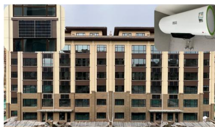
PV electric water heater in Zibo, Shandong Province
