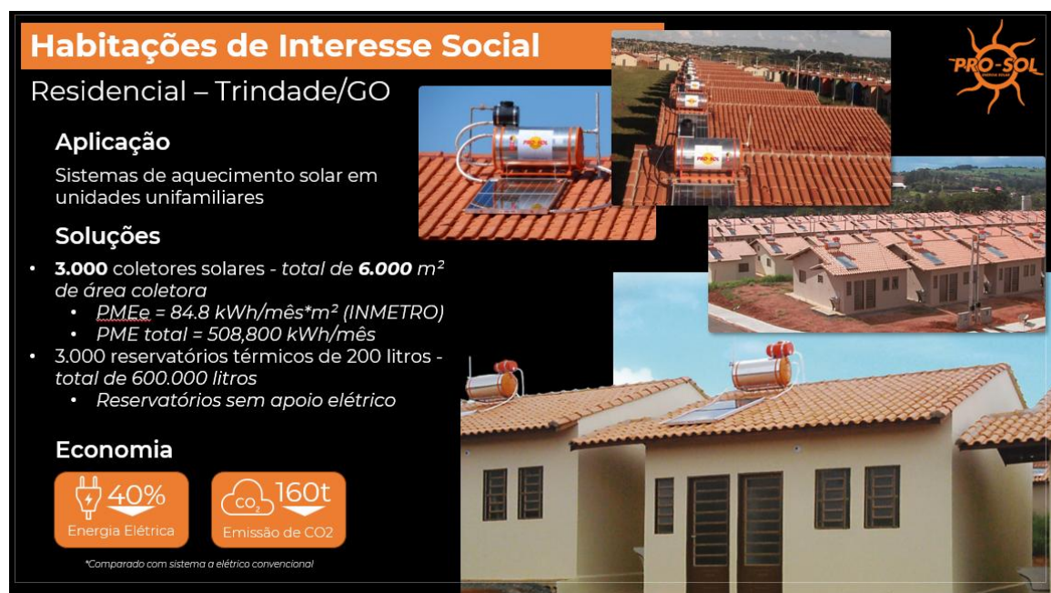
Figure 10. Thermosiphon systems at Social Housing in Trindade, Brazil. Source: Abrasol / Danielle Johann
