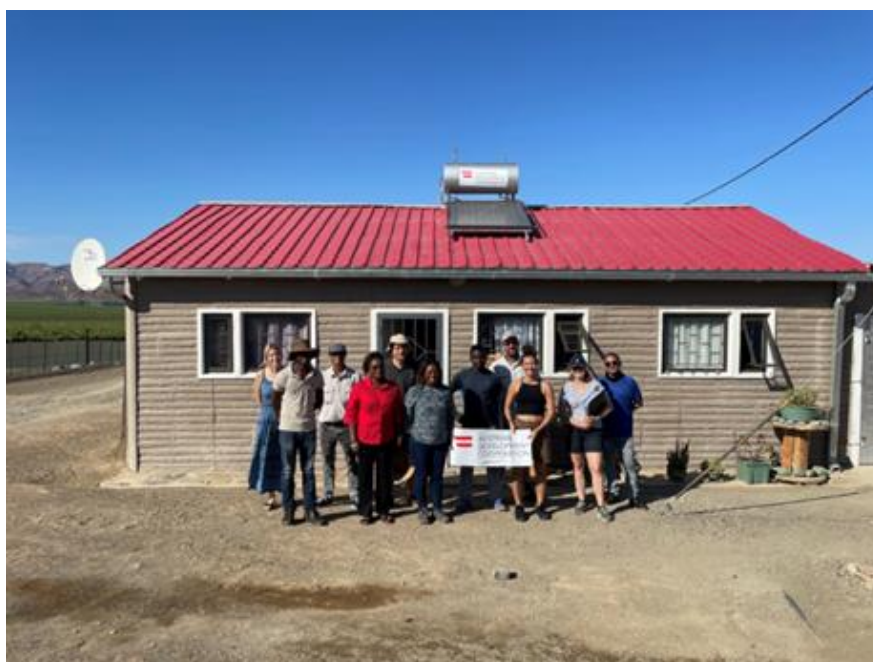
Figure 18. Each house for the vineyard workers is equipped with a solar thermosiphon system. Source: SOLTRAIN
