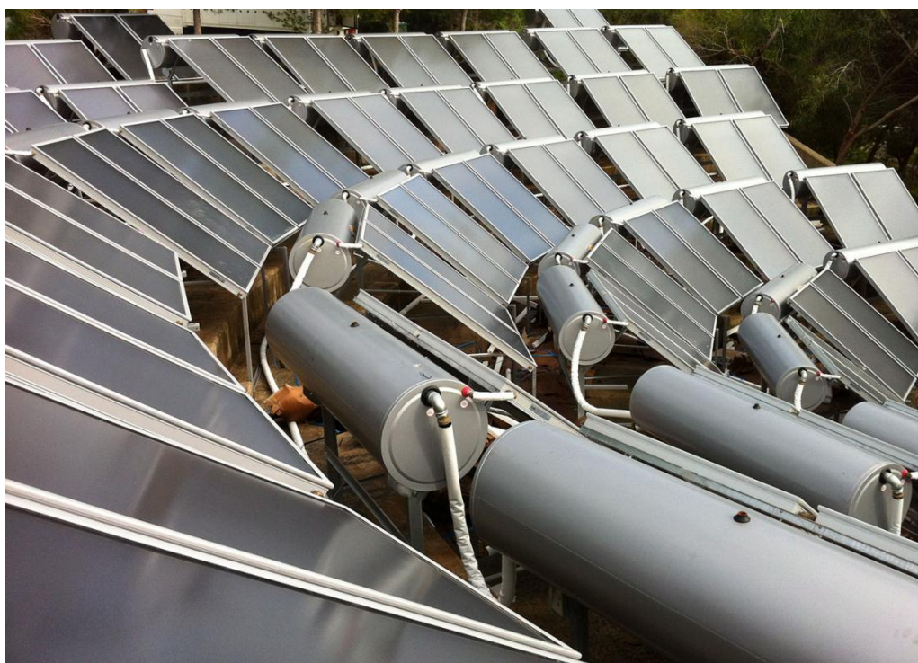
Figure 9. 280 m 2 and 21,000 lt solar thermosyphon system at the Bay Hotel, Zakynthos (Greece). Source: Sole SA https://www.sole.gr/erga#&qid=1&pid=22
