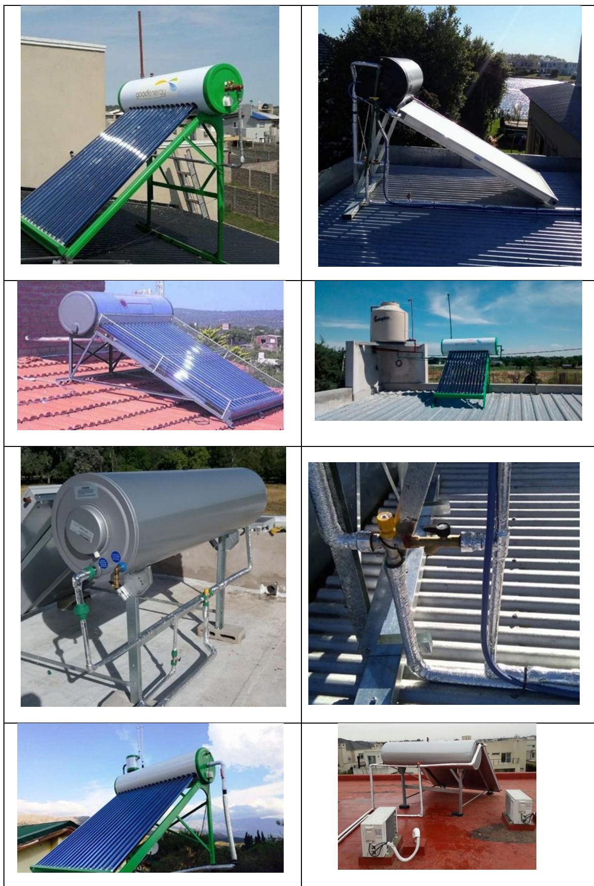
Figure 13. Pictures of common practice thermosiphon systems in Argentina. Photos: Christian Navntoft / Solarmate SA
