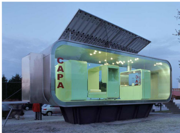
Figure 10. CAPA, Matosinhos, Portugal, 2003. The PV generator is shaped as a sloped plane that characterizes the image of the building. Design: Cannatà & Fernandes. Picture ©Cannatà & Fernandes
