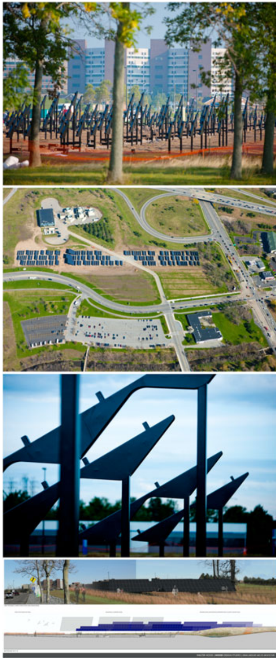
Figure 18. The Solar Strand, Buffalo University Campus, Buffalo (US), 2011. The PV modules on the ground are arranged according to a DNA pattern. They give form to a public space in a direct functional and visual relationship with the buildings of the campus. Design: Walter Hood, Hood Design. Pictures by courtesy of the architect ©W. Hood.
