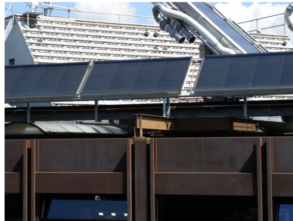
Solar collector field ( T_{\text{solar}} )
