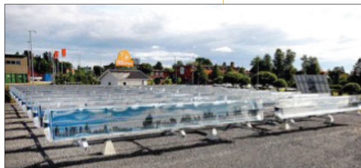
▲ Figure 4. 200 m 2 solar heating collectors installed in Härnösand Energy Park, providing electricity (20 kWp,el) and district heating (80 kWp, th). Source: Absolicon
