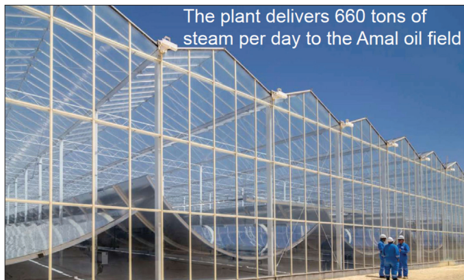
Indoor parabolic trough collectors at the Mirah plant in Oman. Photo credit: Barbara Soldera, GlassPoint Solar, Inc.
