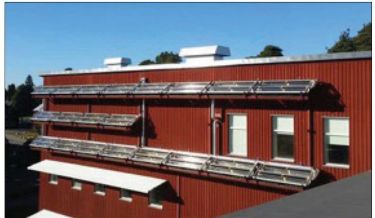
▲ Figure 5. A hybrid PVT installation on a building at the University of Gävle provides electricity (5 kWp, el) and district heating (25 kWp, th) with twenty collectors. Source: Solarus
