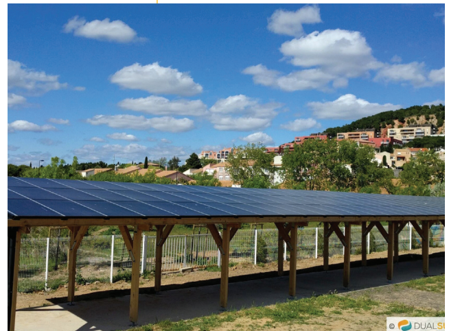
PVT system in the southern French town of Sète supplies heat and electricity to a public pool.
