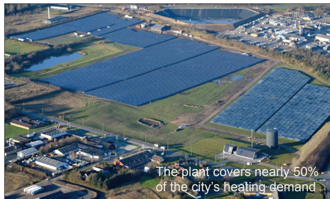
Solar district heating plant with load-balancing pit storage in Vojens, Denmark.
